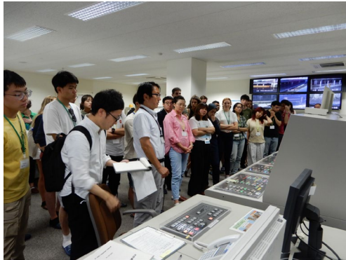
Monitor the movement of the regulating reservoir
