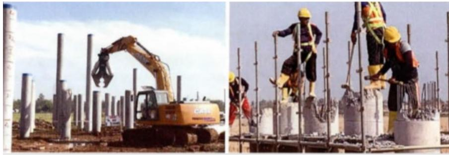
The utilization of Guzzila Concrete Crusher will both increase productivity and make the construction safer
