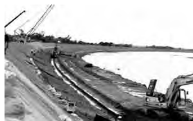
Fig.3 Constructing Mega dike in Pampanga
